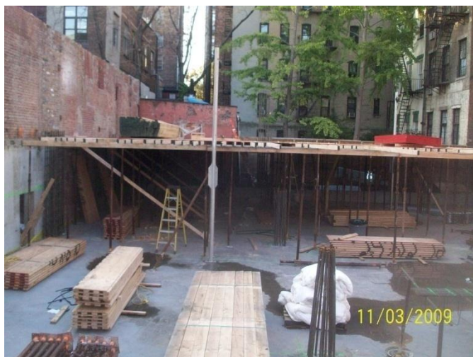
Figure 5: Shows limited material handling due to the space required for shoring and formwork
