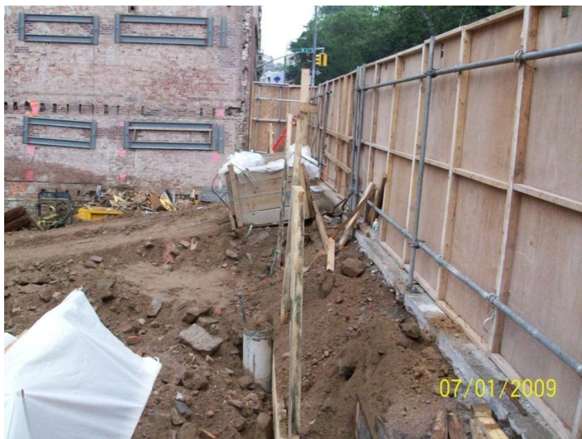
Figure 1: Shows the C-Channel used to reinforce north side of adjacent structure
