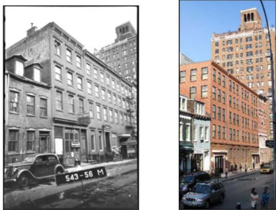
Figure 9: Shows the Pre-1940's Renovation on the Left and the New Project X Building on the Right.
