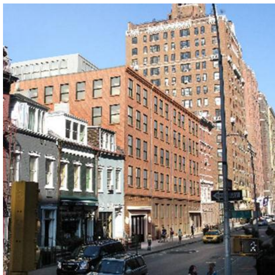
Figure 7: Shows the Adjacent Height Restrictions and the Metal façade Used on the Roof Level.
