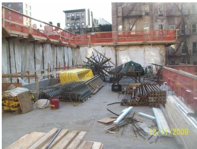
Figure 4: Illustrates the Very Limited Storage Area
