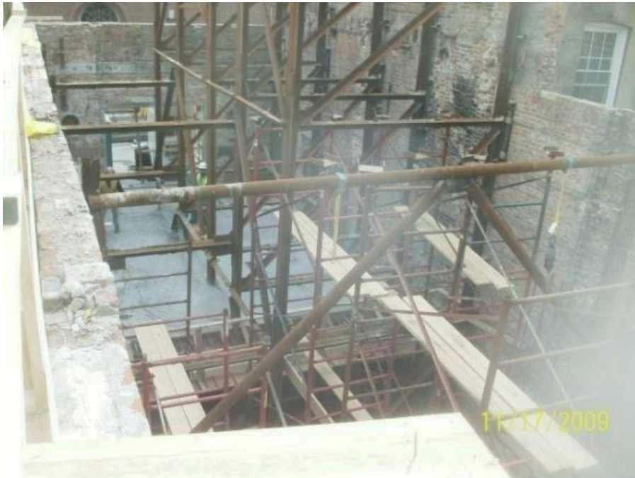
Figure 3: Shows an Up-close View of the Structural Steel Bracing
