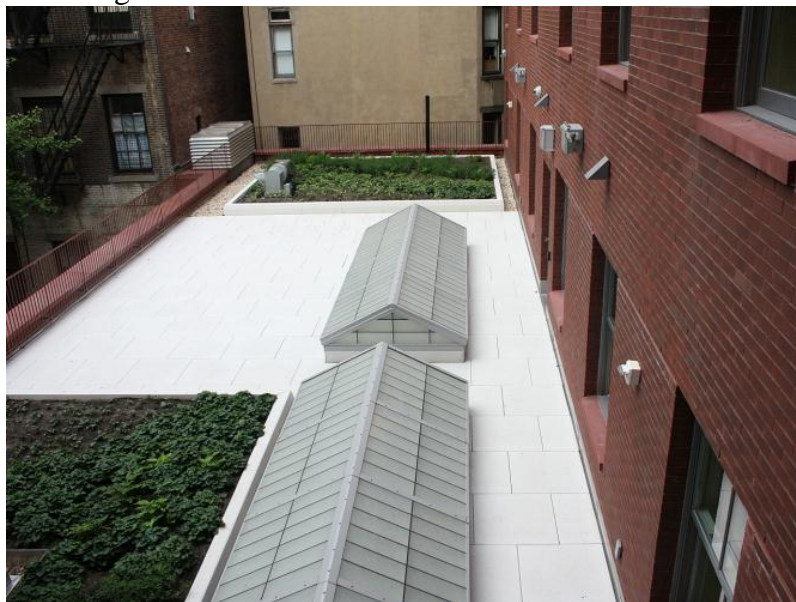
Figure 8: Shows Green Roof and Aluminum Railing
